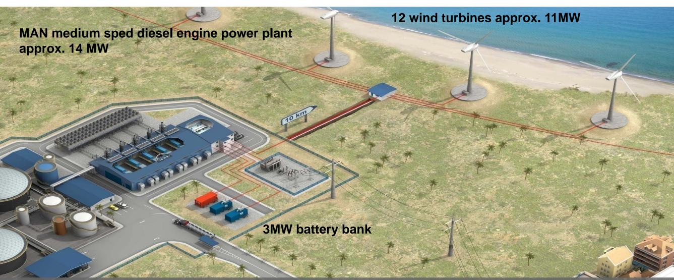
The world's largest wind and diesel power plant in Bonaire supplies up to 25 MW environmentally friendly energy for the island's 15,000 inhabitants.
